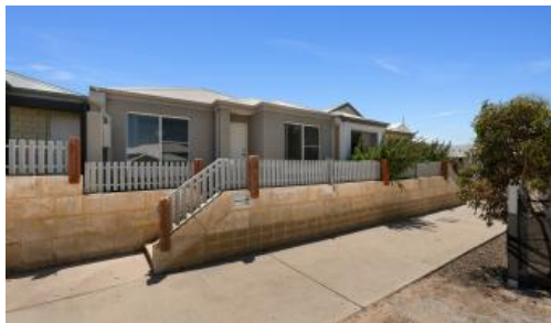
256 Shorehaven Blvd, Alkimos
